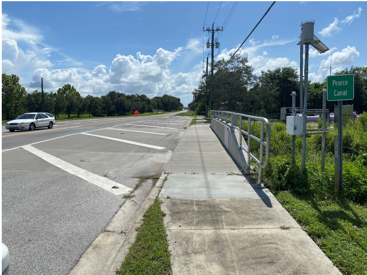
Figure 19: Bridge Over Pearce Canal (looking east)
