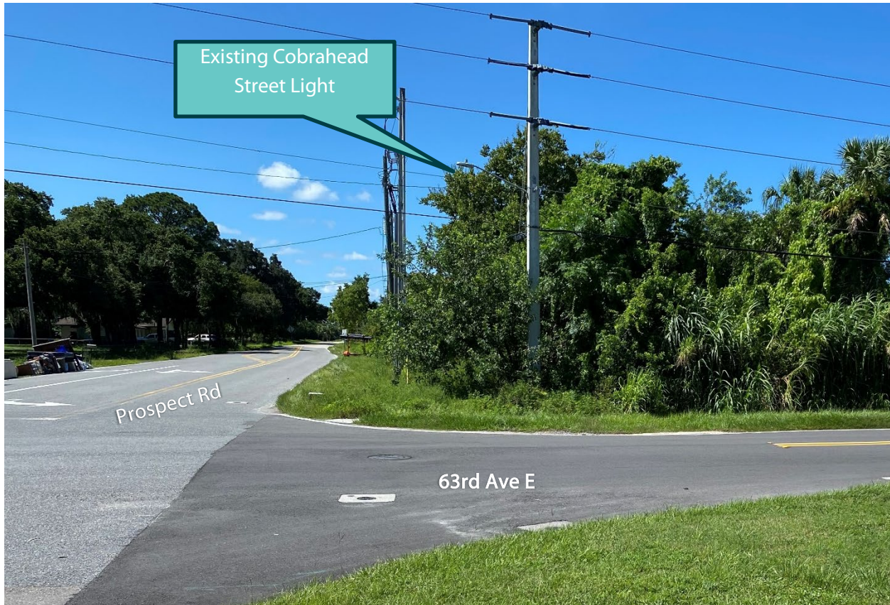
Figure 15: Existing Street Light (looking south)
