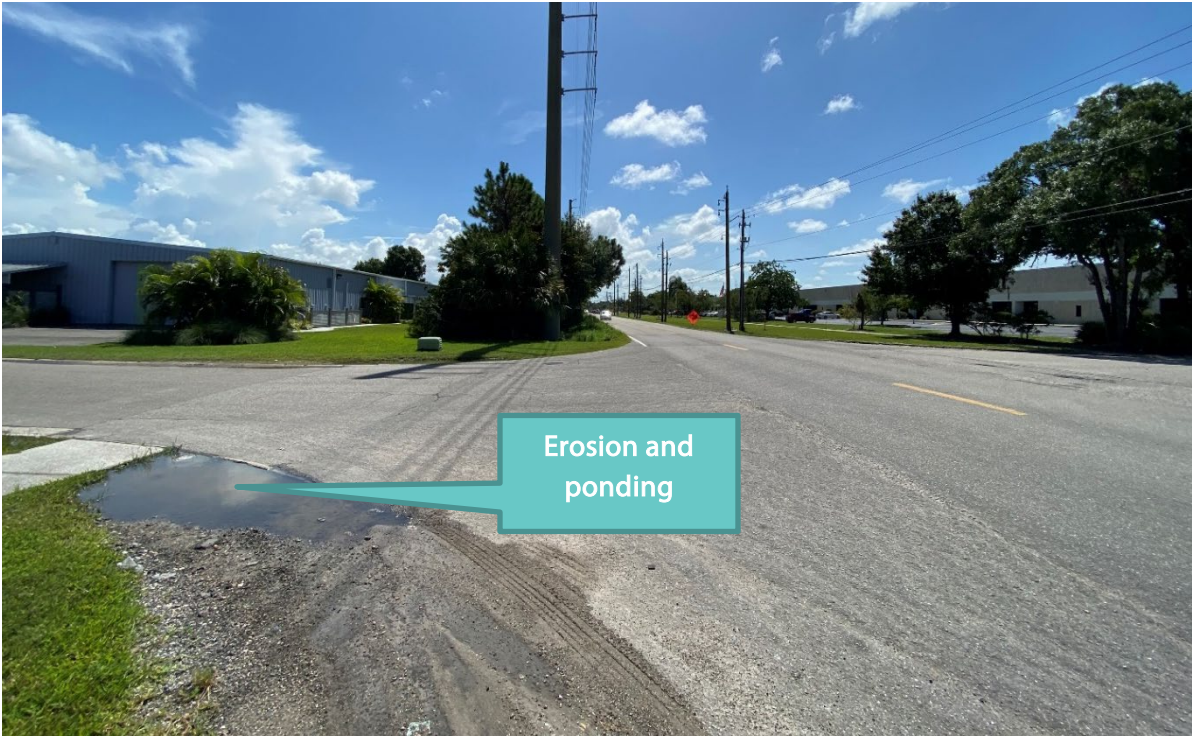
Figure 22: Erosion Around Side of Weir (looking north)
