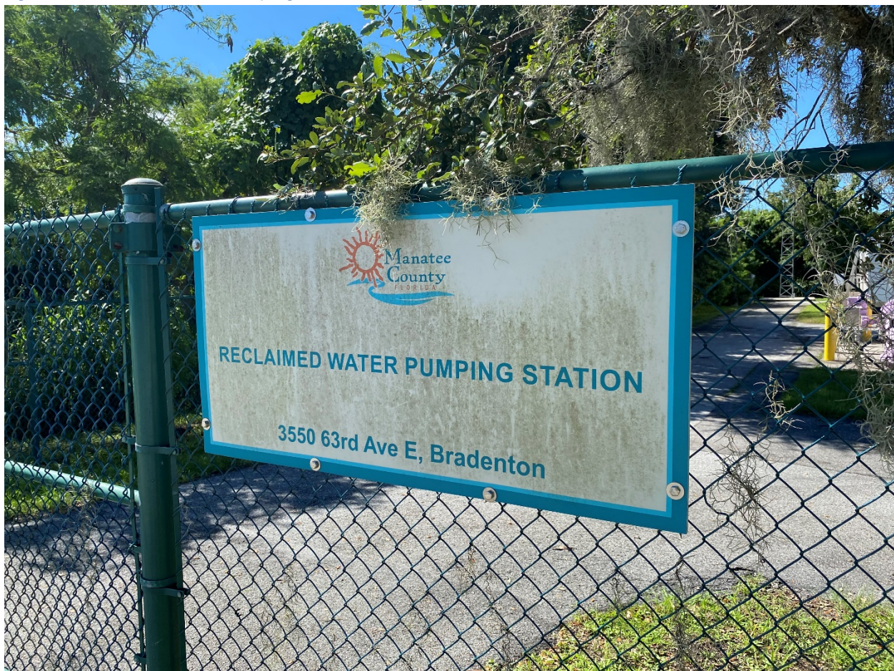
Figure 17: Reclaimed Water Pumping Station (looking south)
