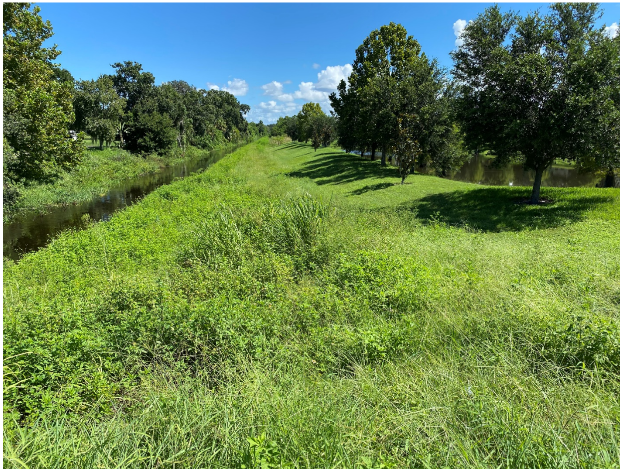
Figure 3: Pearce Canal (looking north)
