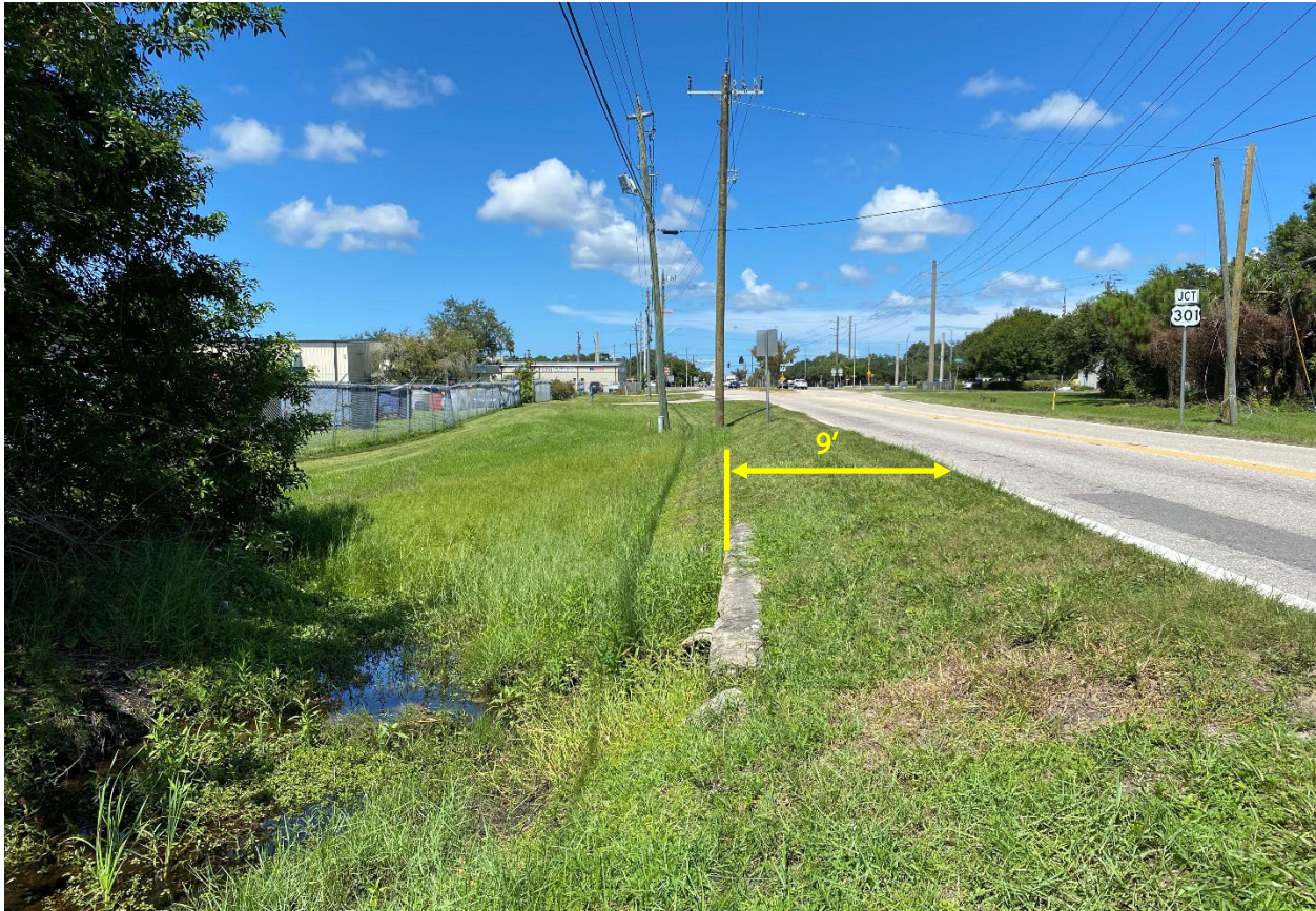
Figure 12: Endwall in the Clear Zone of 63rd Avenue (looking west)
